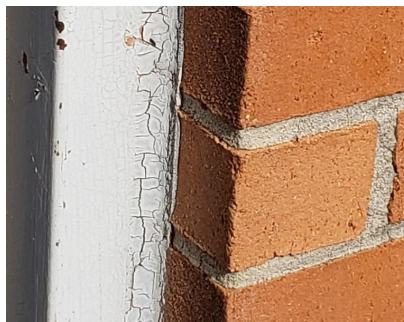
Sealant deterioration
