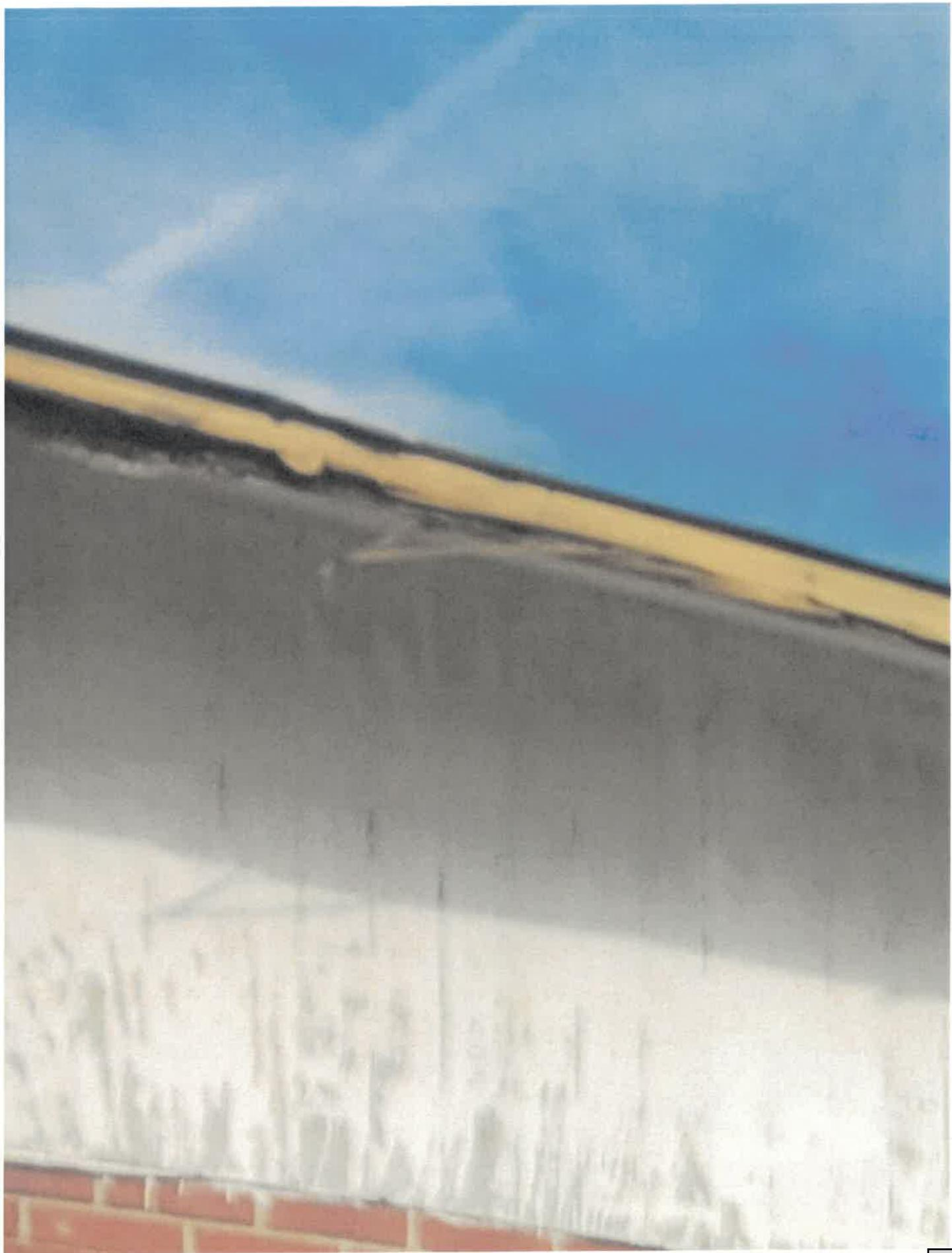
Complete roof removal, the under original roof is flat concrete and is in good condition so going back to that Historic look on entire roof .
