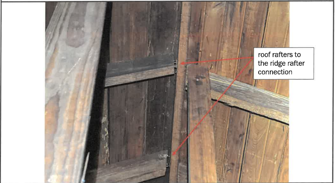
Photo 4: Failed connection at ridge rafter
