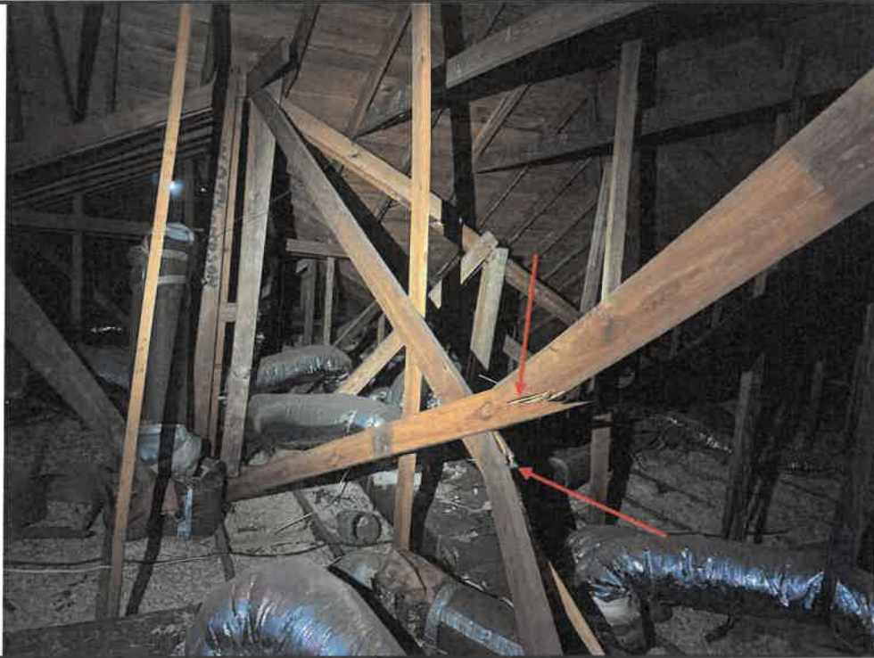
Photo 5: Broken x-bracing between Truss-A and Truss-B
