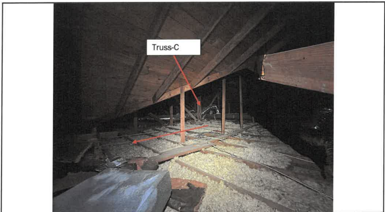
Photo 7: Attic view – Attic joists and bottom chord of the Truss-C slopping toward north
