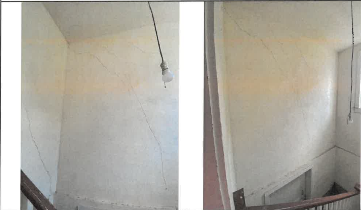
Photo 8: Cracks on the walls – Signs of marginal differential settlement and absence of a bond beam at the top of the wall.
