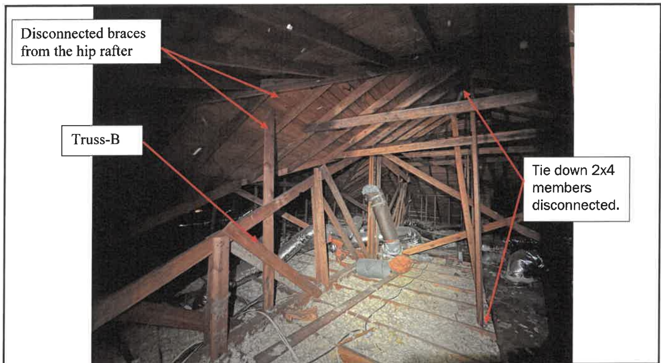
Photo 1: Attic view – Main Truss-B
