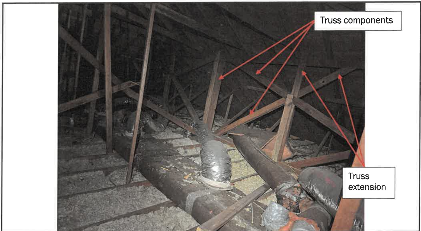
Photo 3: Attic view – Truss-A
