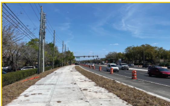
ALTAMONTE SPRINGS MOBILITY PLAN SR 436 - WALKING & TRANSIT IMPROVEMENT UNDER CONSTRUCTION
