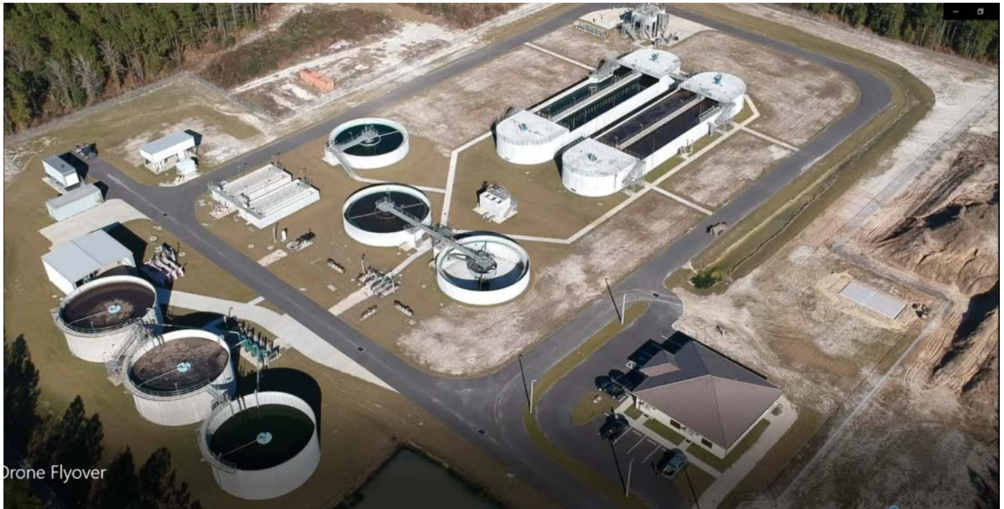
Drone Flyover Kicklighter Wastewater Treatment Plant
