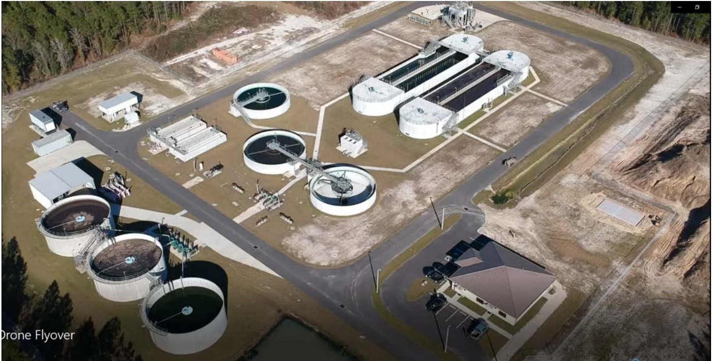
Drone Flyover Kicklighter Wastewater Treatment Plant
