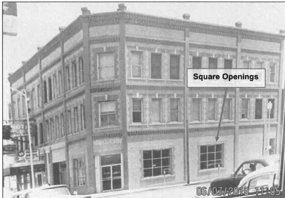
Photo 2: Building with Modifications
