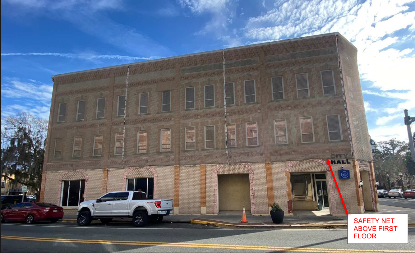
Photo 1: West Building Face
