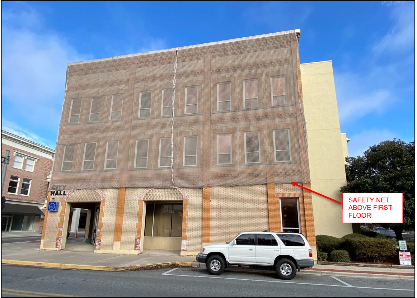
Photo 2: South Building Face
