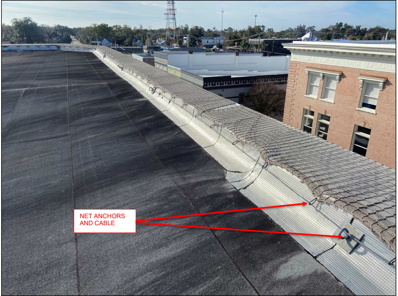
Photo 4: Net Anchors on Roof Parapet
