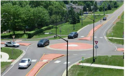
Example of a single-lane roundabout. Source: FHWA
