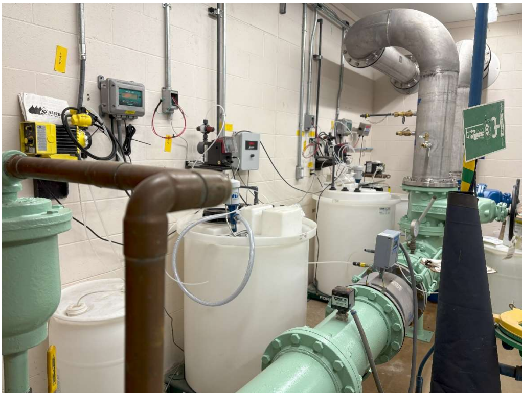
Chemical Feed Equipment Installed
