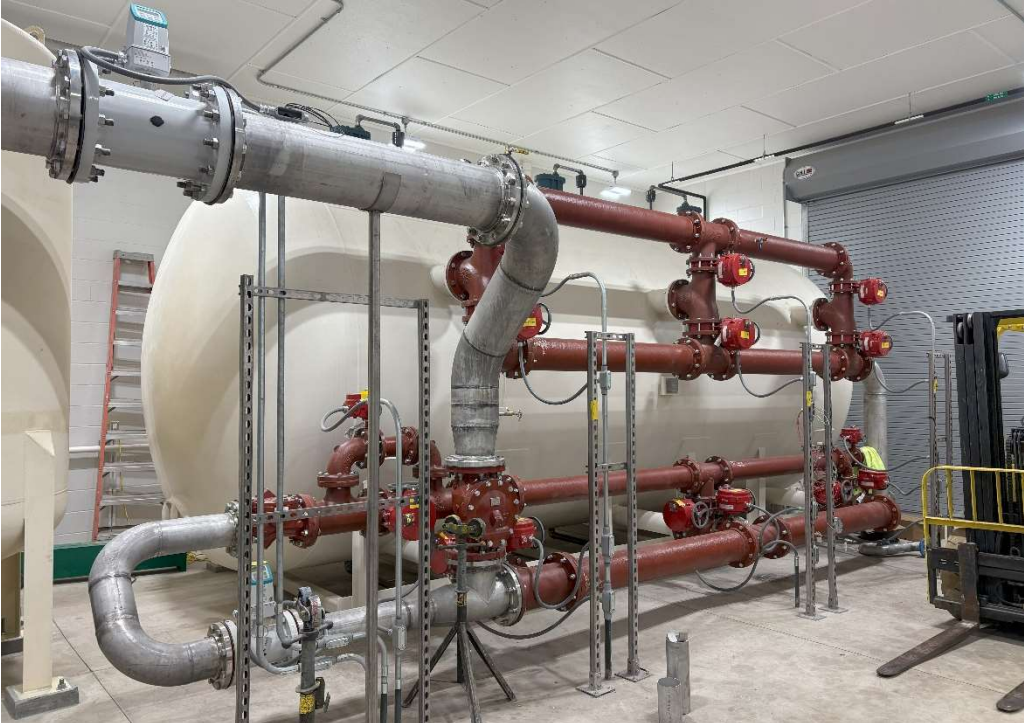
Process Piping Installed
