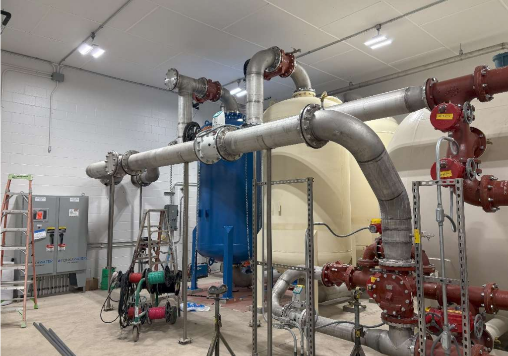
Process Piping Installed
