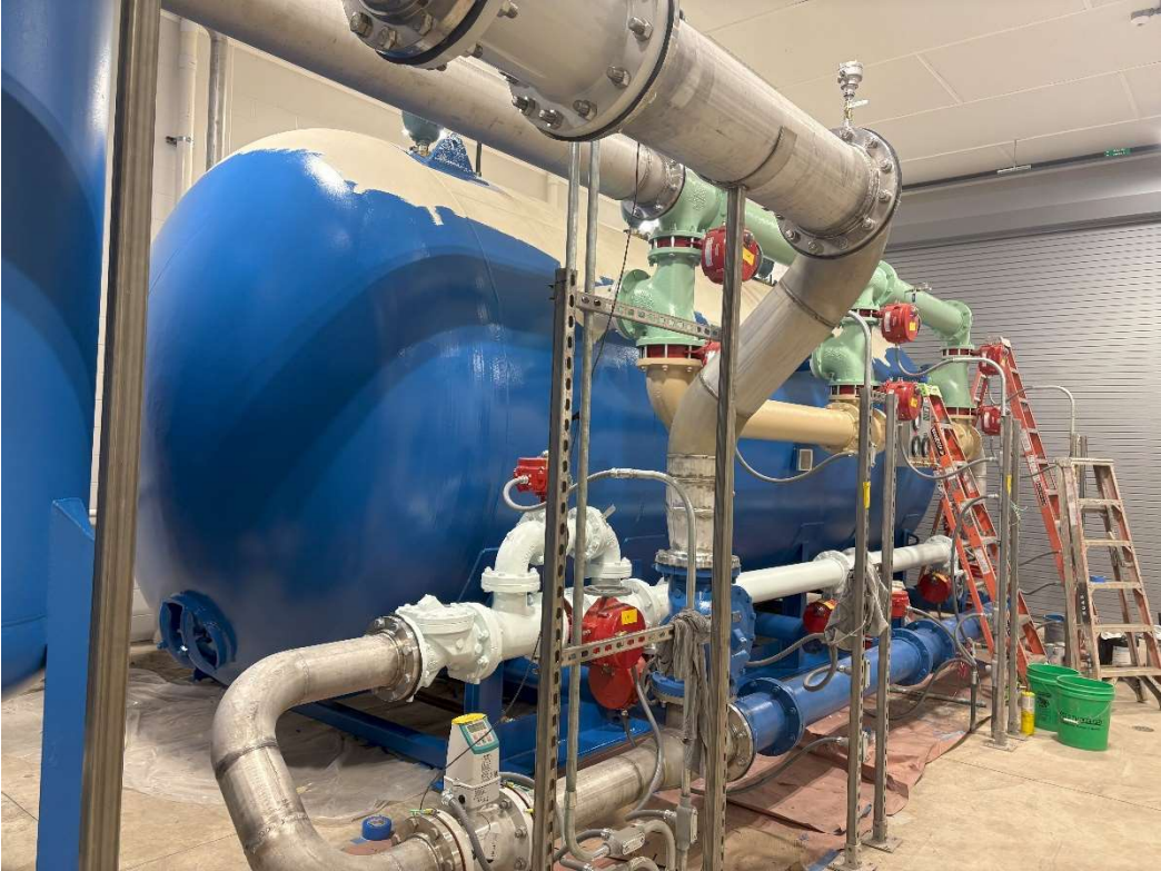
Final Coat of Paint on Horizontal Vessel
