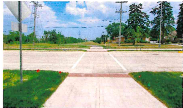
SOUTH 68TH STREET CONCRETE REPLACEMENT GREENFIELD, WI
