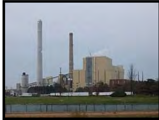
WPS Weston Power Plant
