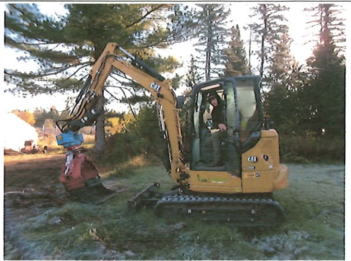
Cat 304 Excavator Operated by Vinnie Tesch
