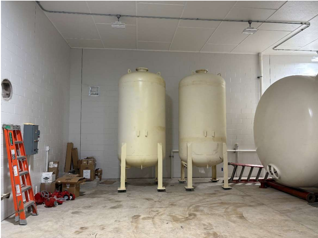
2 Vertical Vessels Installed
