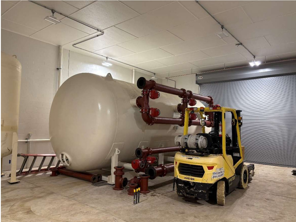
Horizontal Pressure Vessels With Piping Manifold Piping Started
