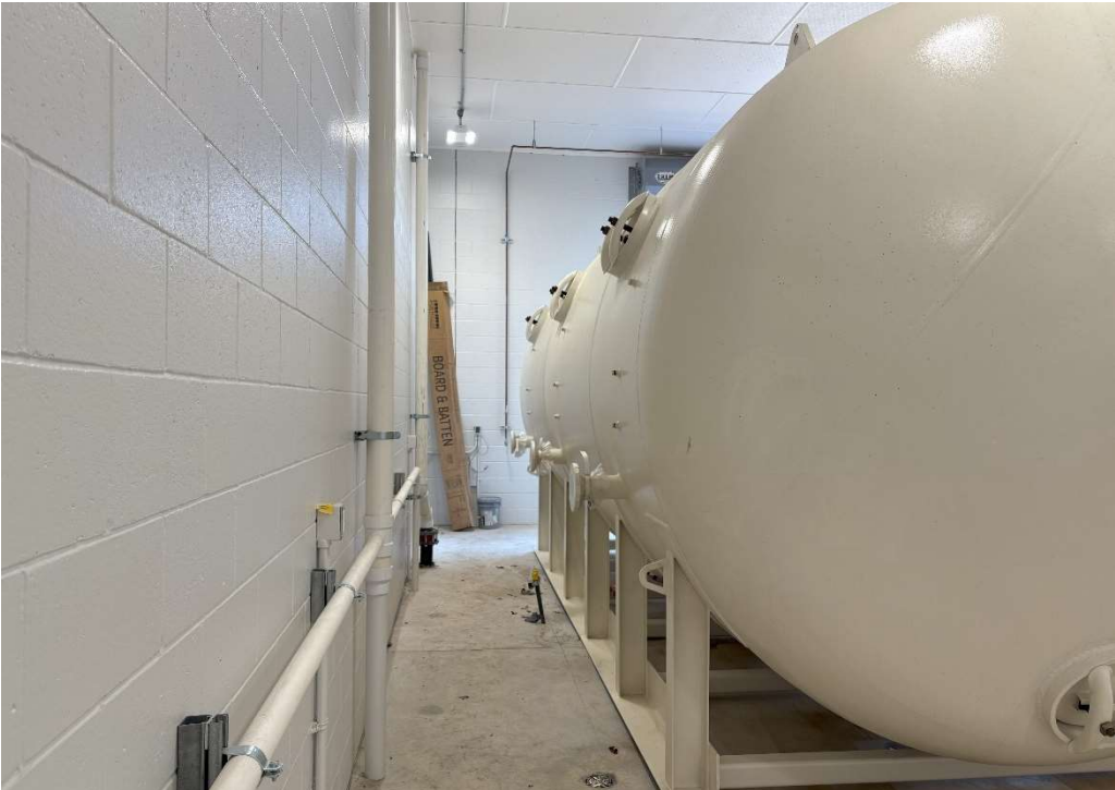
North Side of Pressure Vessel
