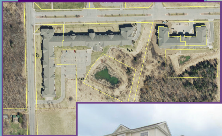
EXAMPLE: Birchwood Highlands Apartments 8005 Birch Street, Weston, WI, 54476
