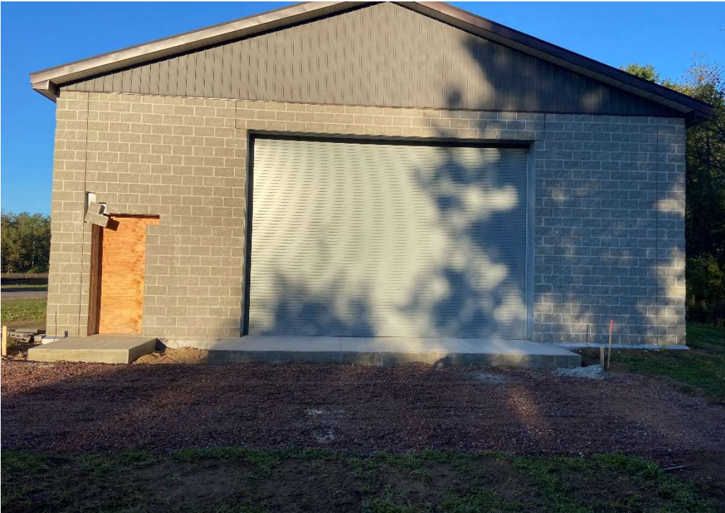
Overhead Door Installation and Approach Slab Finish
