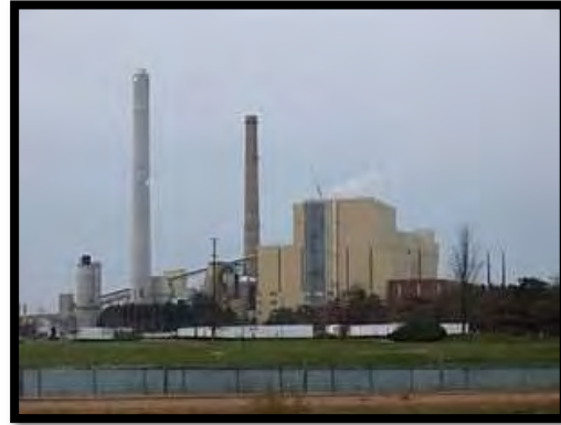
WPS Weston Power Plant
