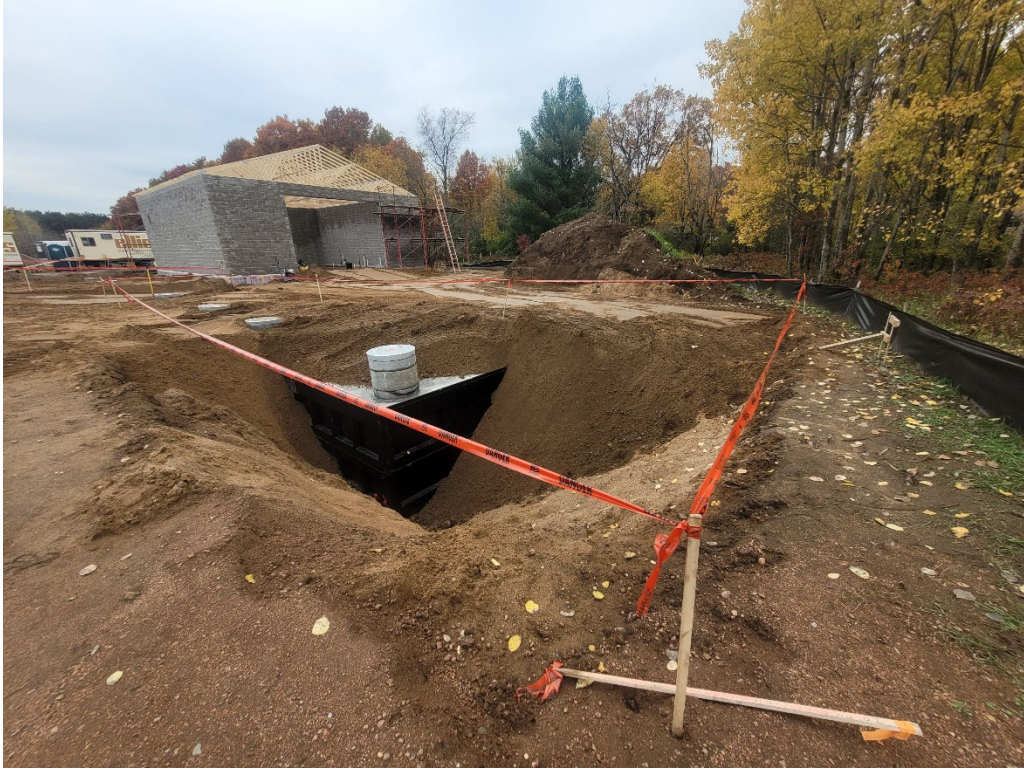
Underground tanks backfilled, trusses installed
