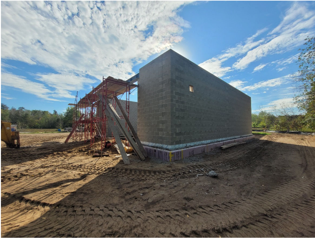
8" Concrete Masonry Unit Wall, at northeast corner
