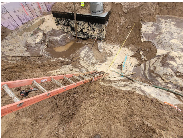
Excavation Hole after Water Pumped Out
