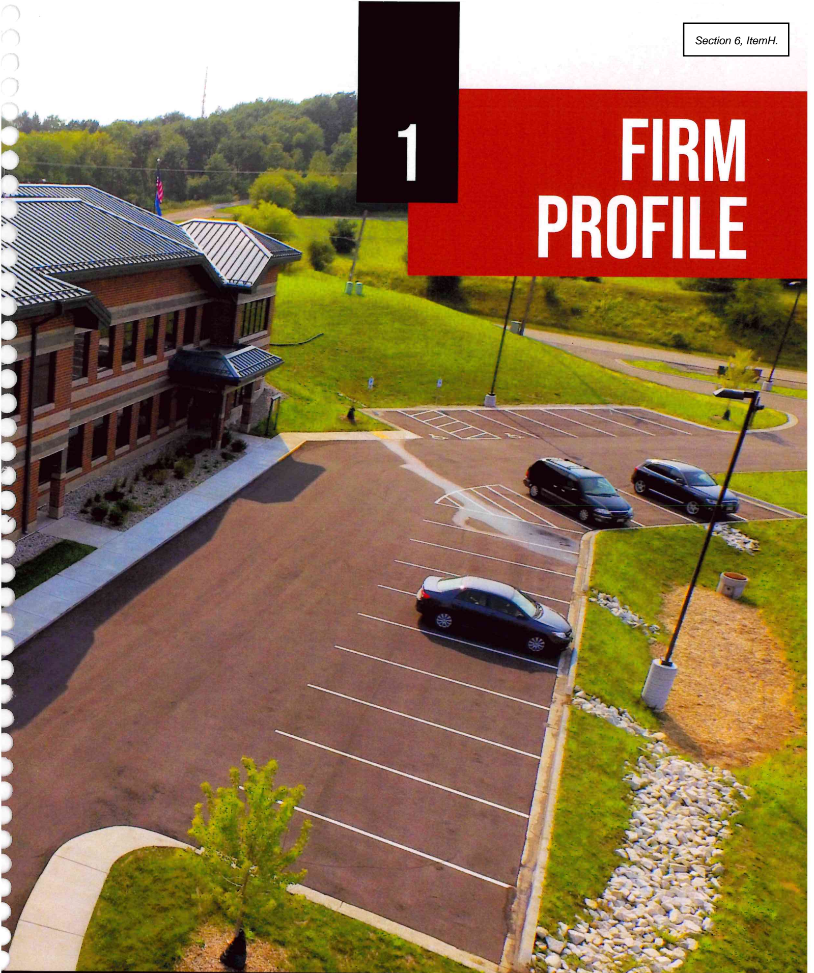
Delafield Fire Station Delafield, W
