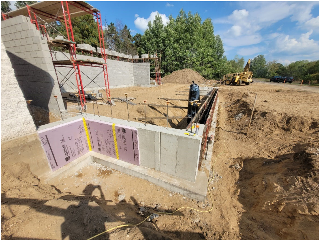
Footings, frost walls, and concrete masonry walls
