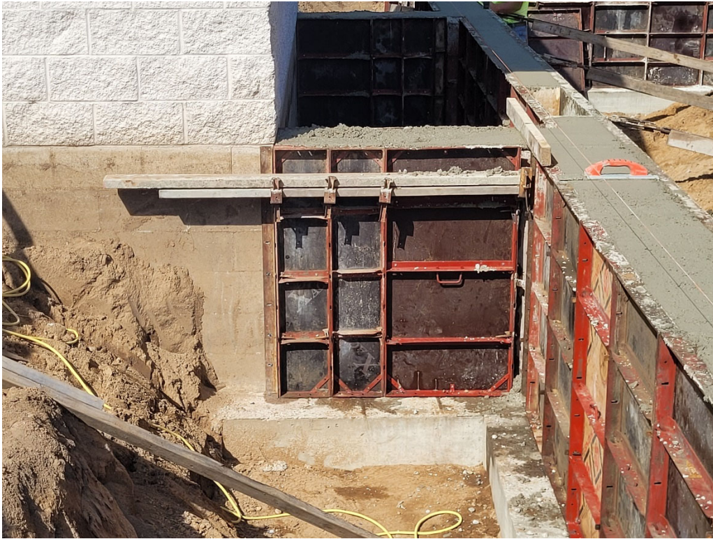
Footings and frost wall at southeast corner Well #2
