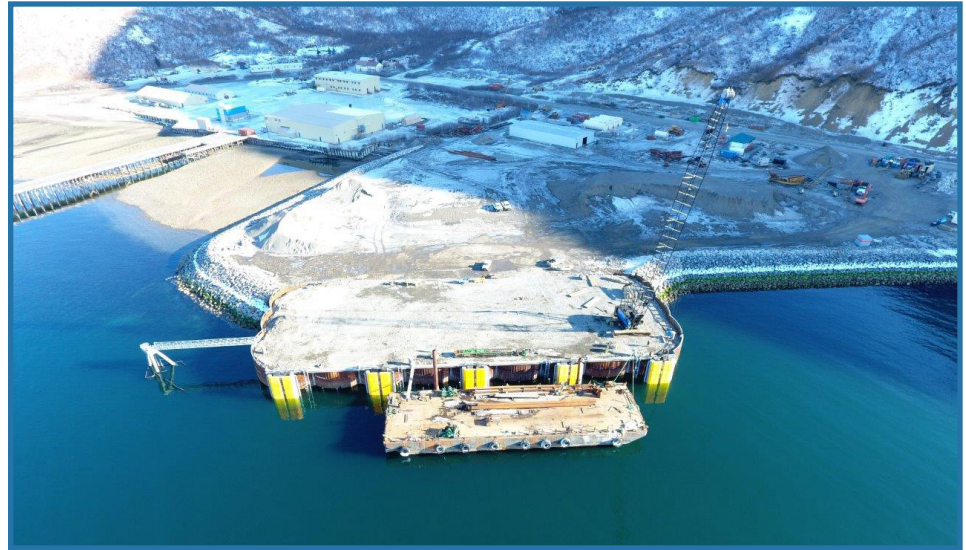
Chignik Dock (under construction)
