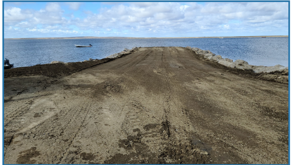
Chefornak Temporary Barge Landing (under construction)
