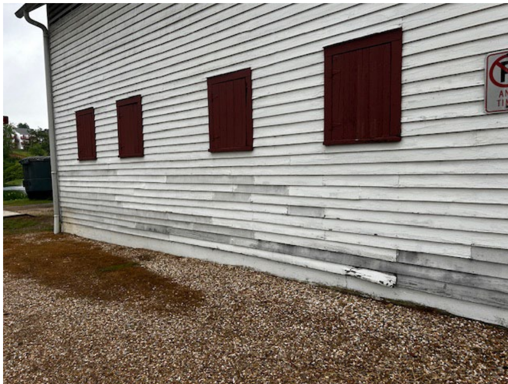
Harvey Barn – Area showing rotted boards and deterioration of paint.
