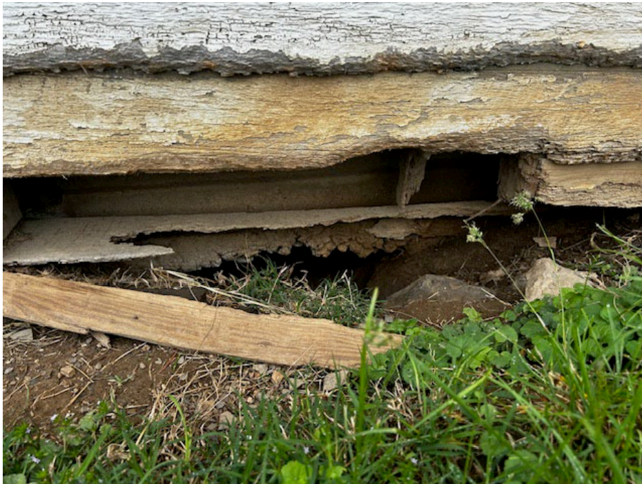
Bathroom Building: Photo of rotting boards at bottom of building and foundation failure.
