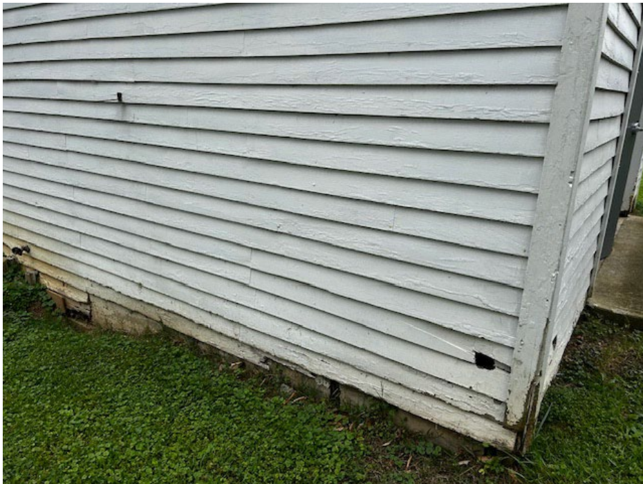
Bathroom Building: Photo of rotting boards at bottom of building and foundation failure.
