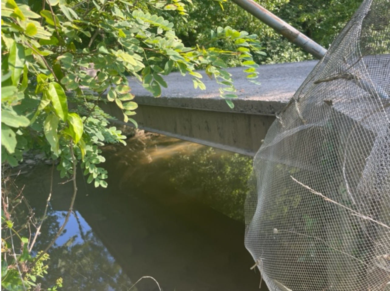
Existing bridge over Horse Creek
