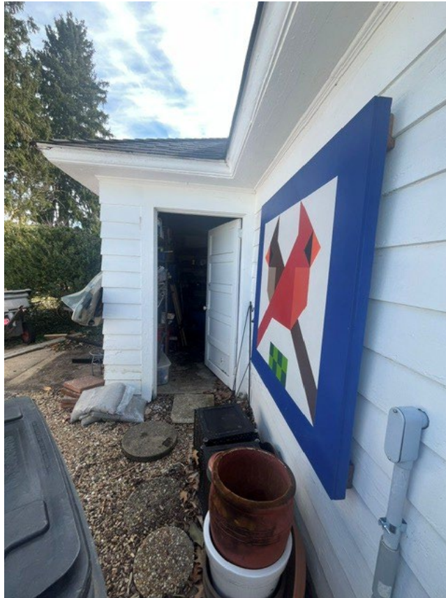
Storage shed at the rear of the garage—requested for demolition and removal.
