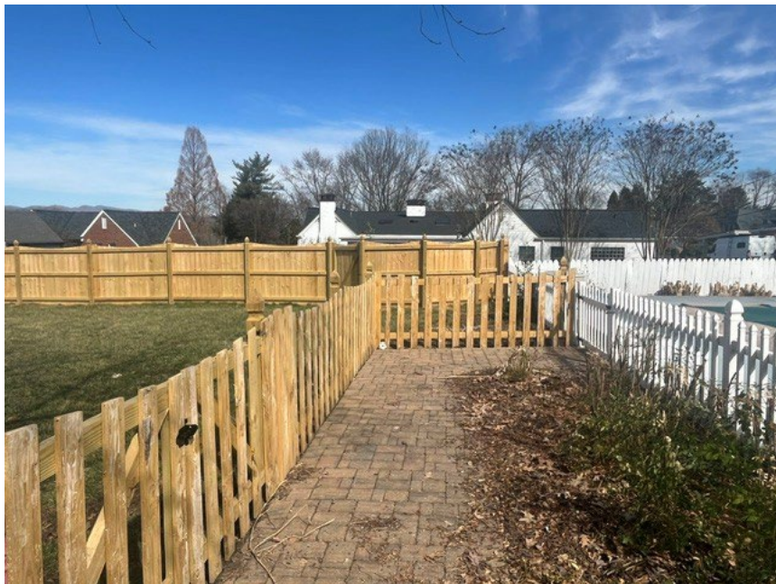
A photo of the approved fencing, approved in November 2024, which will replace the existing pool fencing.
