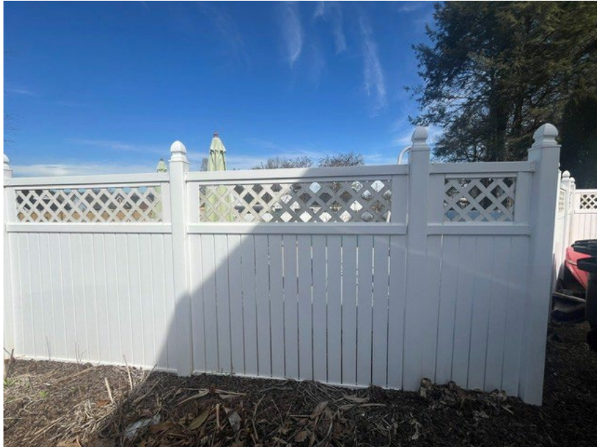
Existing fencing at 1236 Watauga Street—set to be removed and replaced.
