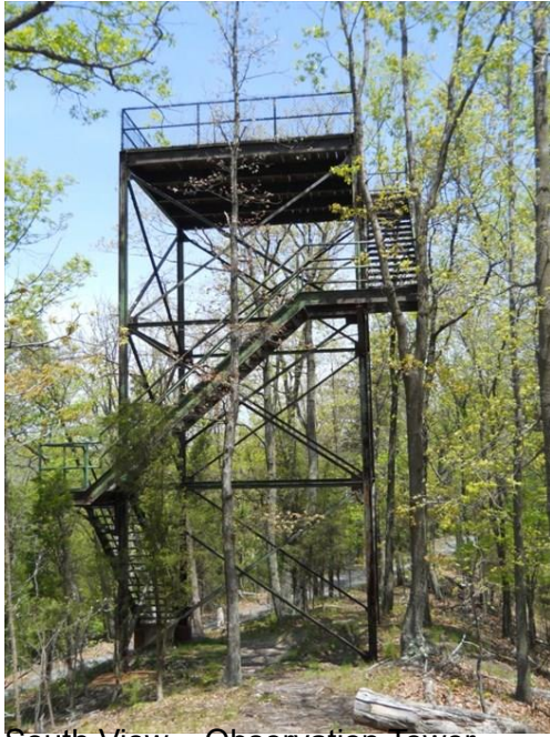
South View – Observation Tower
