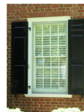
The original twelve-over-twelve, wood sash window at 1261 Watuga Street reflects the dwelling's Colonial Revival style.
