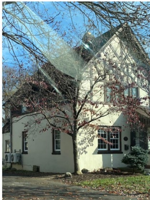
House view after window in front and on left side were replaced.
