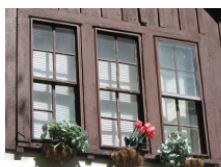
Original four-over-four, wood sash windows at 205 Compton Terrace.
