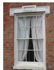
This original six-over-six, wood-sash window with ornamental hood is an important component of Rotherwood.
