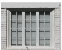
Original casement windows at 809 Yarkin Street.
