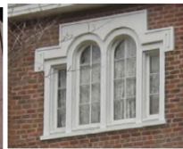
Rotherwood features this variation of a Classical Palladian window.
