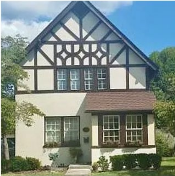
Picture of house before two windows on left were replaced. Please note Entryway windows on the right will not be replaced. Also, when approved all windows (8) on the top floor will be replaced. House paint also needs to be touched up and will be done with approved paint colors.
