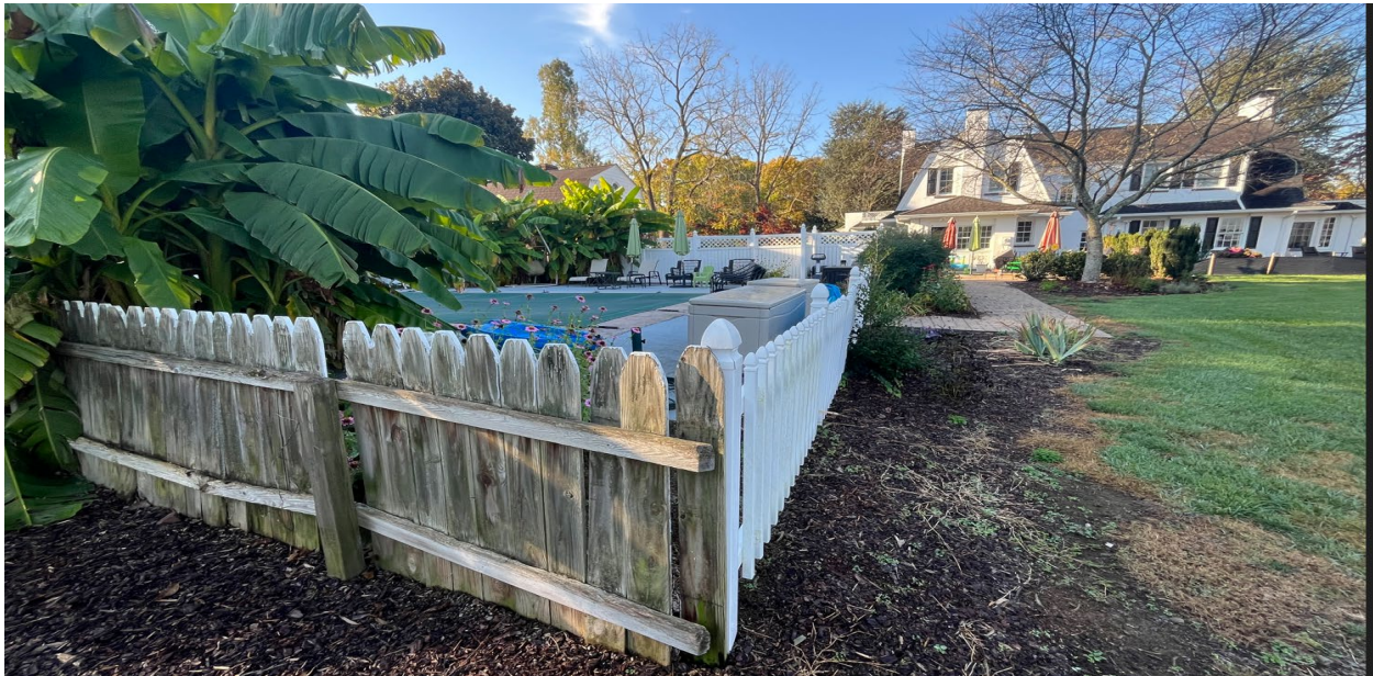
Rear yard view facing south, illustrating the connection point for the proposed 6-foot fence
