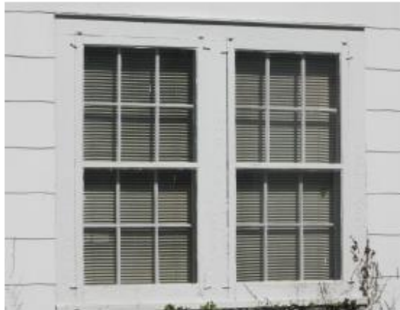
Example of an appropriate wood storm window over original six-over-six wood-sash windows (706 Yadkin Street)
