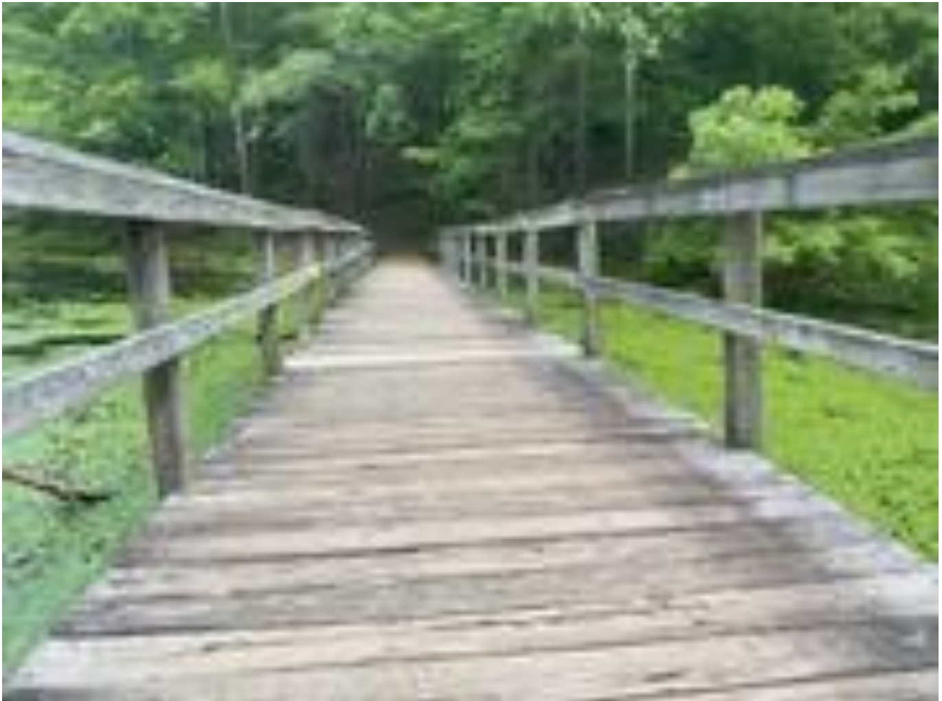
Looking toward the lower Lakeside Trail, the lean in the bridge's structure is visible.
