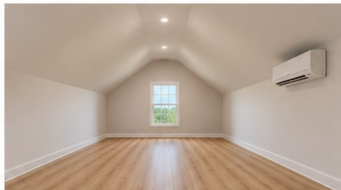
ATTIC – FINISHED WITH SHEETROCK & LVT FLOORING
