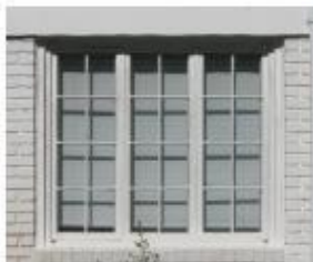
Original casement windows at 509 Yadkin Street.
