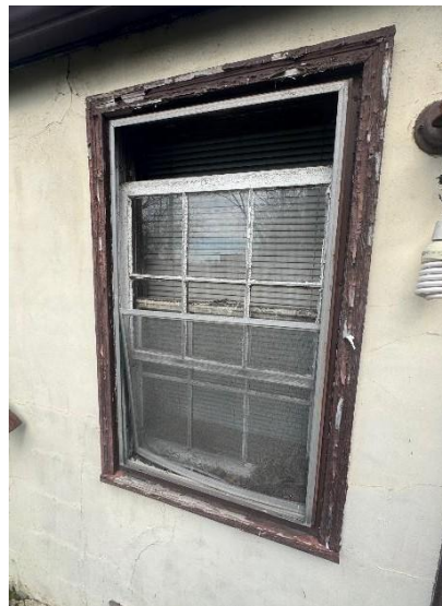
Windows and Gutter on the unit
