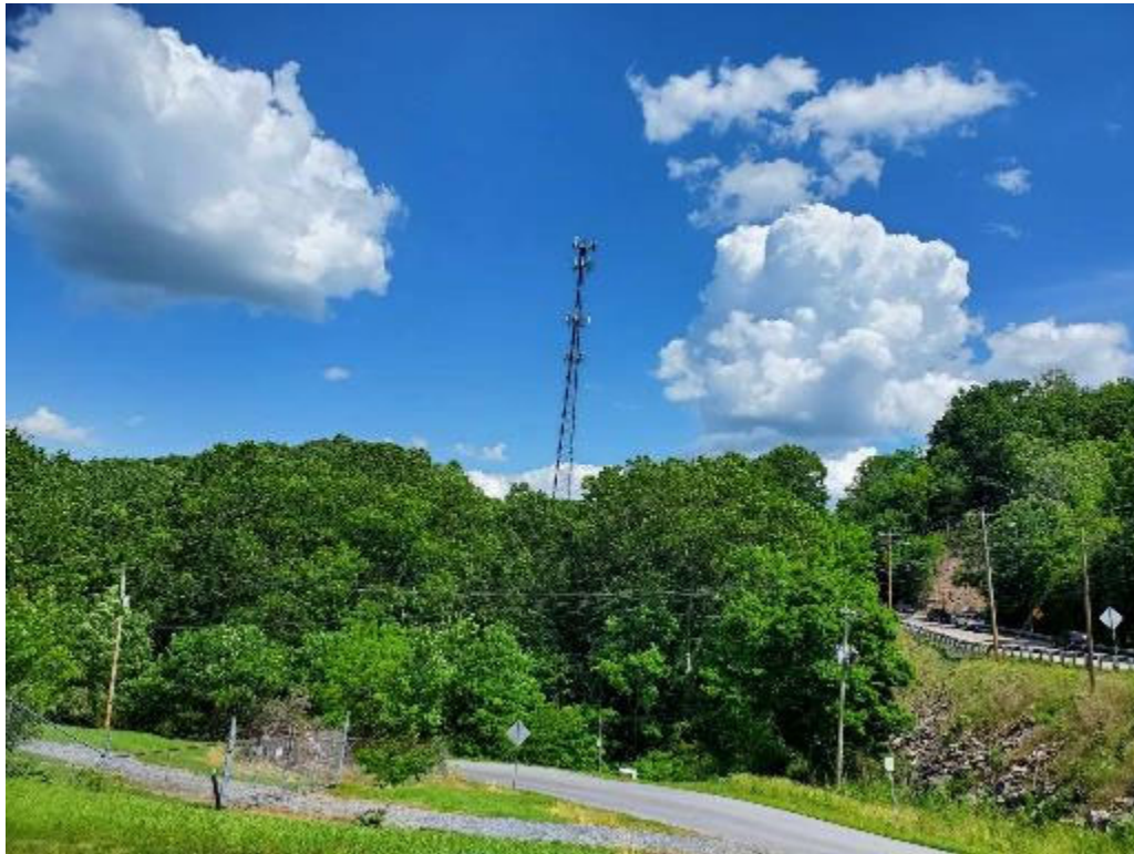
View of Tower from Subdivision Entrance (Lakeside Lane)
