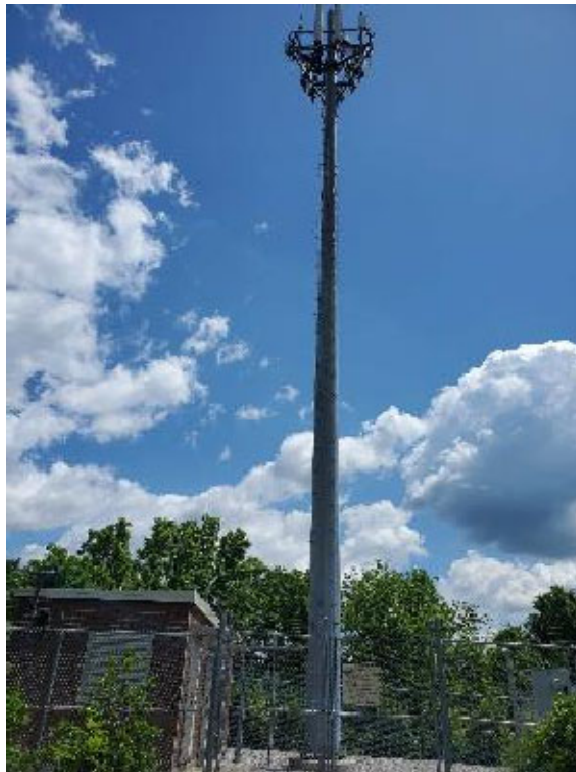
View of Tower
