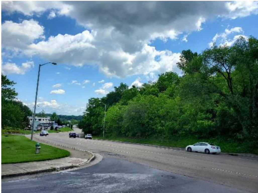
View North Along N. Eastman Road
