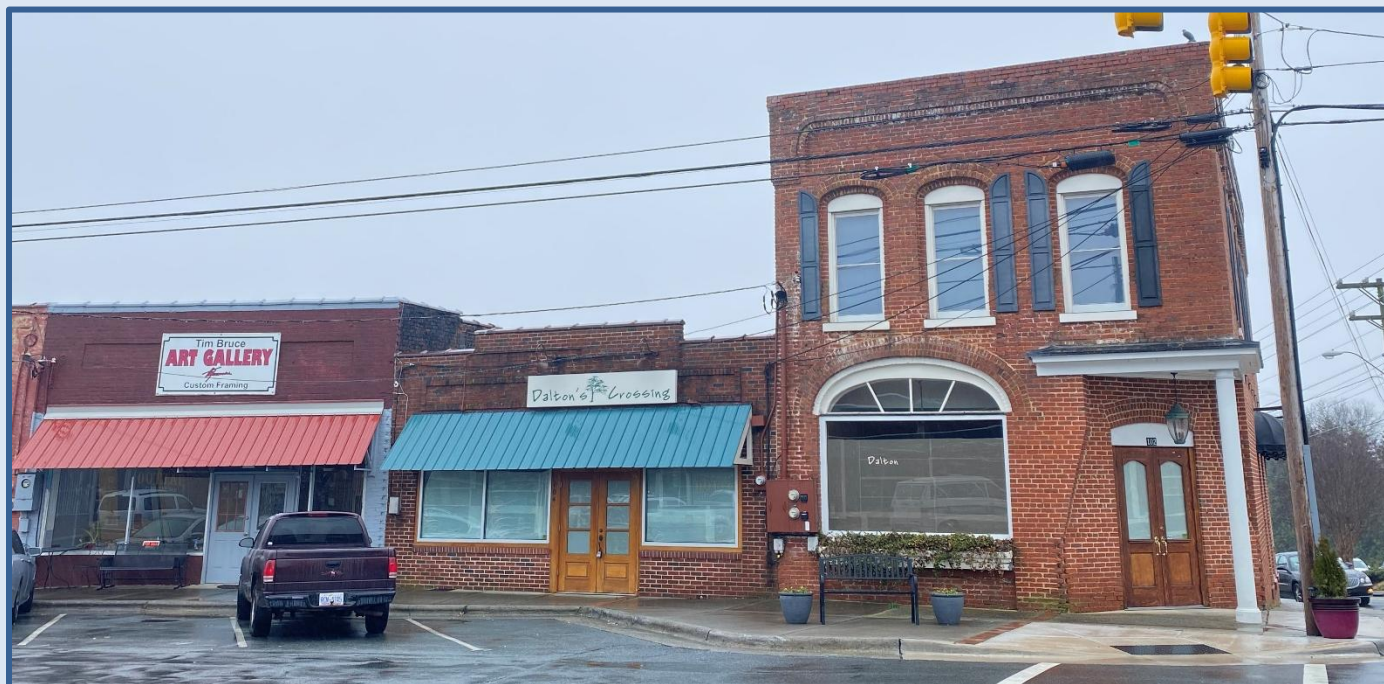
Photo taken by staff from the community site tour in Downtown King on March 3, 2025
