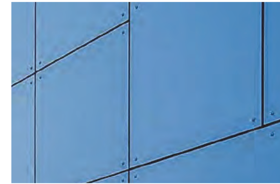
EXTERIOR FINISH 5 (EF-5): SOLID PHENOLIC PANEL RAINSCREEN, STONEWOOD ARCHITECTURAL PANELS, 7875-CB LAPIS BLUE
