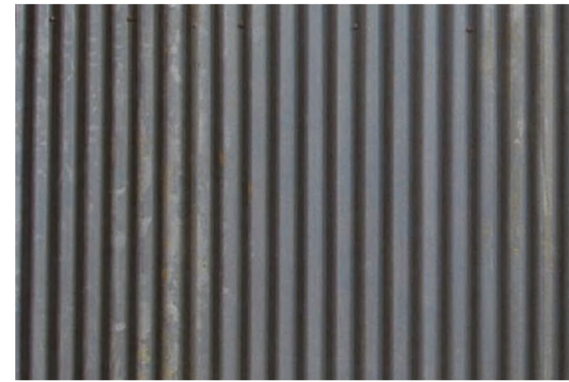
EXTERIOR FINISH 7 (EF-7): CORRUGATED METAL, VERTICAL SIDING, WESTERN STATES METAL ROOFING, MATTE PATINA
