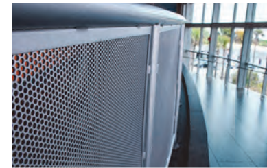
GUARDRAIL 1 (GR-1): MATTE BLACK PERFORATED SHEET METAL
