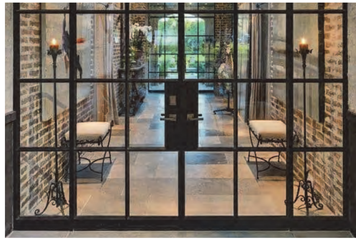
DOORS AND WINDOWS, GROUND FLOOR: BLACK ANODIZED THERMALLY BROKEN ALUMINUM STOREFRONT SYSTEM
