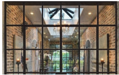
DOORS AND WINDOWS, GROUND FLOOR: BLACK ANODIZED THERMALLY BROKEN ALUMINUM STOREFRONT SYSTEM
