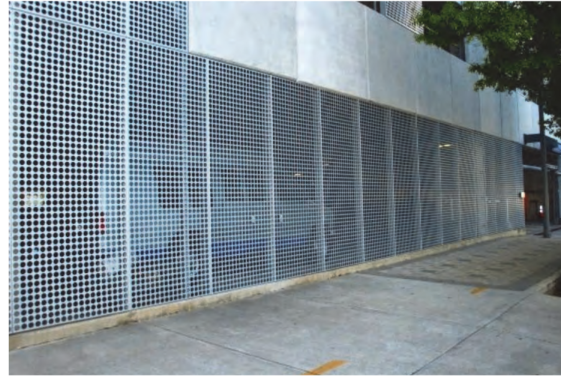
EXTERIOR FINISH 8 (EF-8): PERFORATED SHEET METAL
