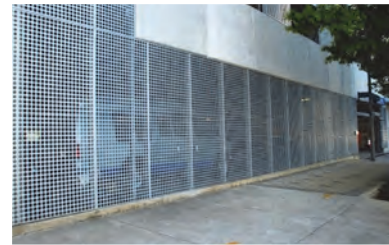
EXTERIOR FINISH 8 (EF-8): PERFORATED SHEET METAL
