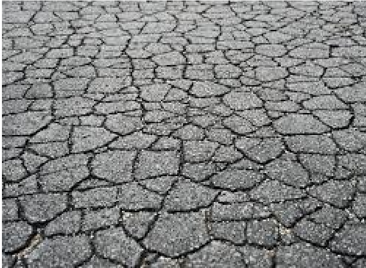
Alligator Cracking
