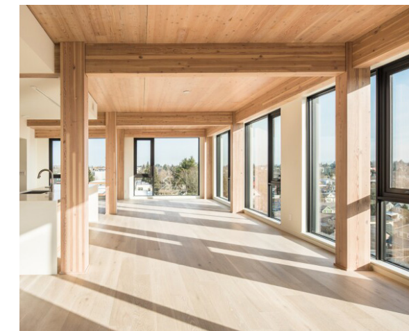
CLT Structure Smartlam, Montana
