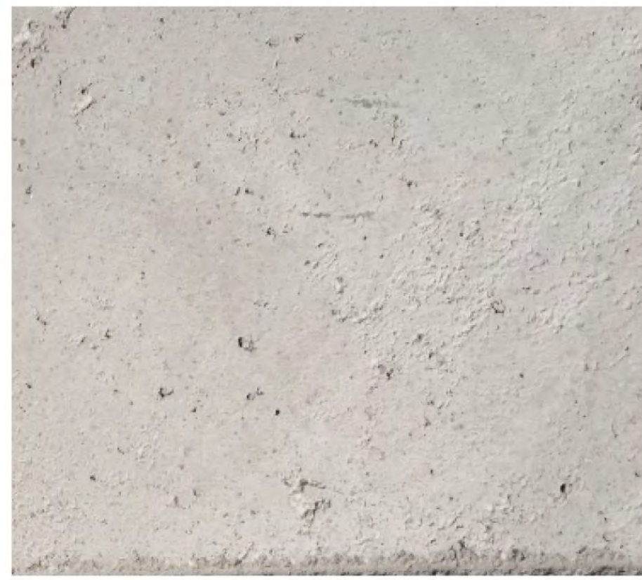
CONCRETE: BASE + STEPS
