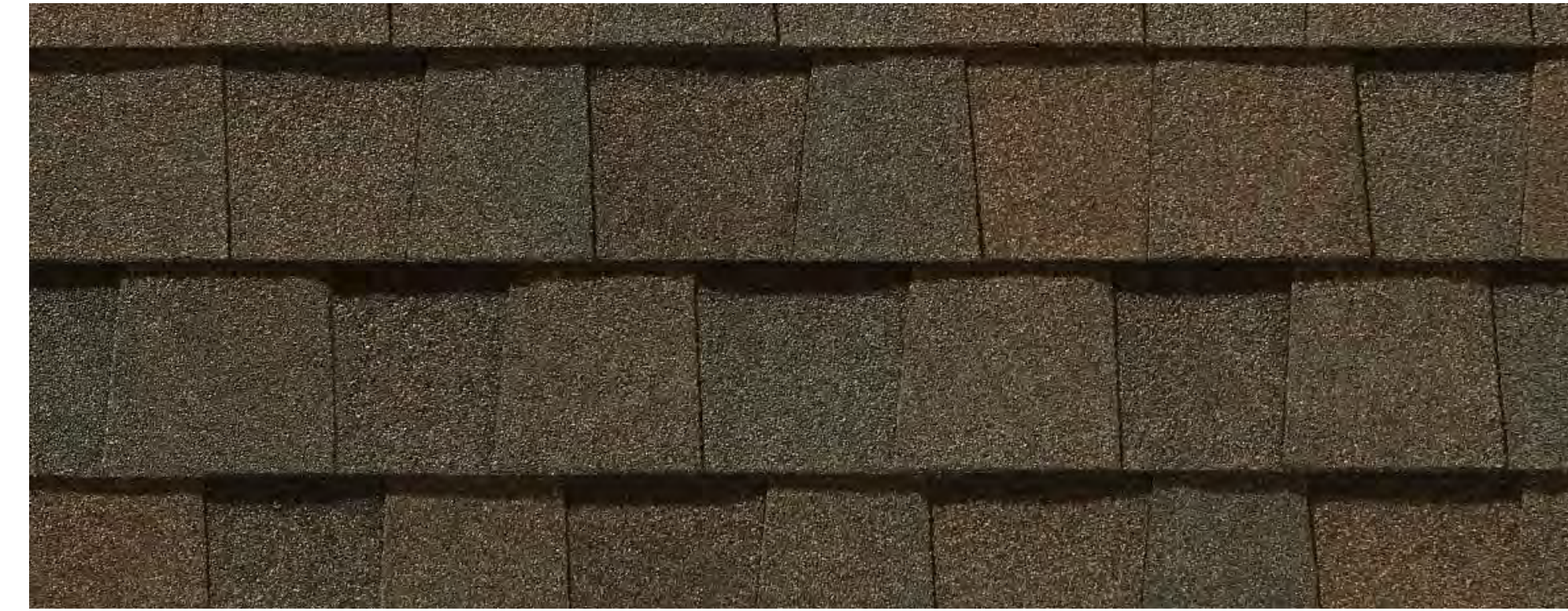
ASPHALT SHINGLE ROOF
