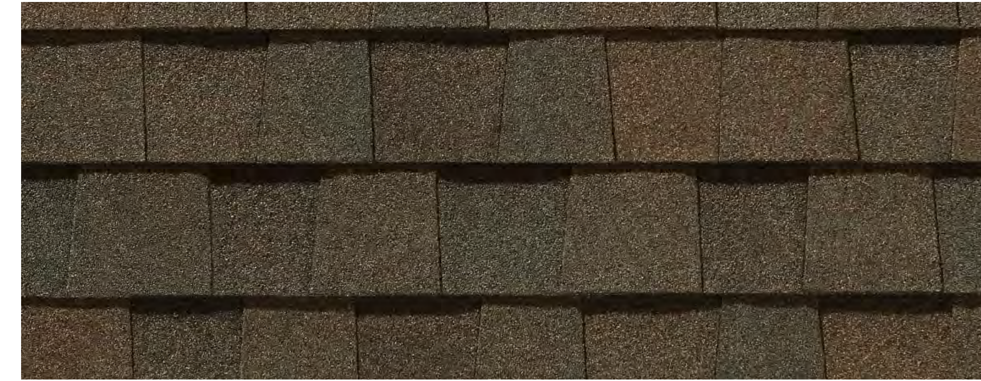
ASPHALT SHINGLE ROOF
