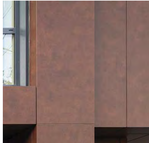
ALUMINUM PANELS with colored and textured FEVE resin-based powder coating system. Basis of Design: Pure + FreeForm coated aluminum panels with Vintage Steel #FA049 / Color Family: Rust finish.
