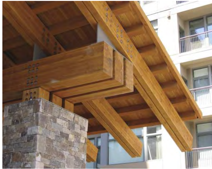
HEAVY TIMBER GLULAM BEAMS, RAFTERS AND COLUMNS with painted galvanized structural steel knife-plate connections. Fasteners to be recessed galvanized steel or stainless steel. Clear heart Western Red Cedar heavy timber purlins and T&G decking with resawn finish. Wood clear coat stain.
