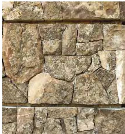
STONE VENEER - Montana Moss Rock natural stone dry-stack lay-up. Stainless steel masonry anchor system.
