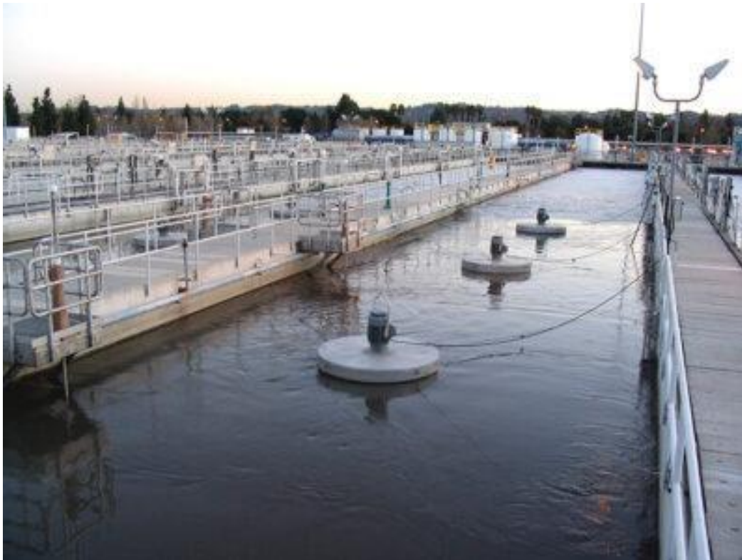
Figure 2. Example of a Floating Mixer
