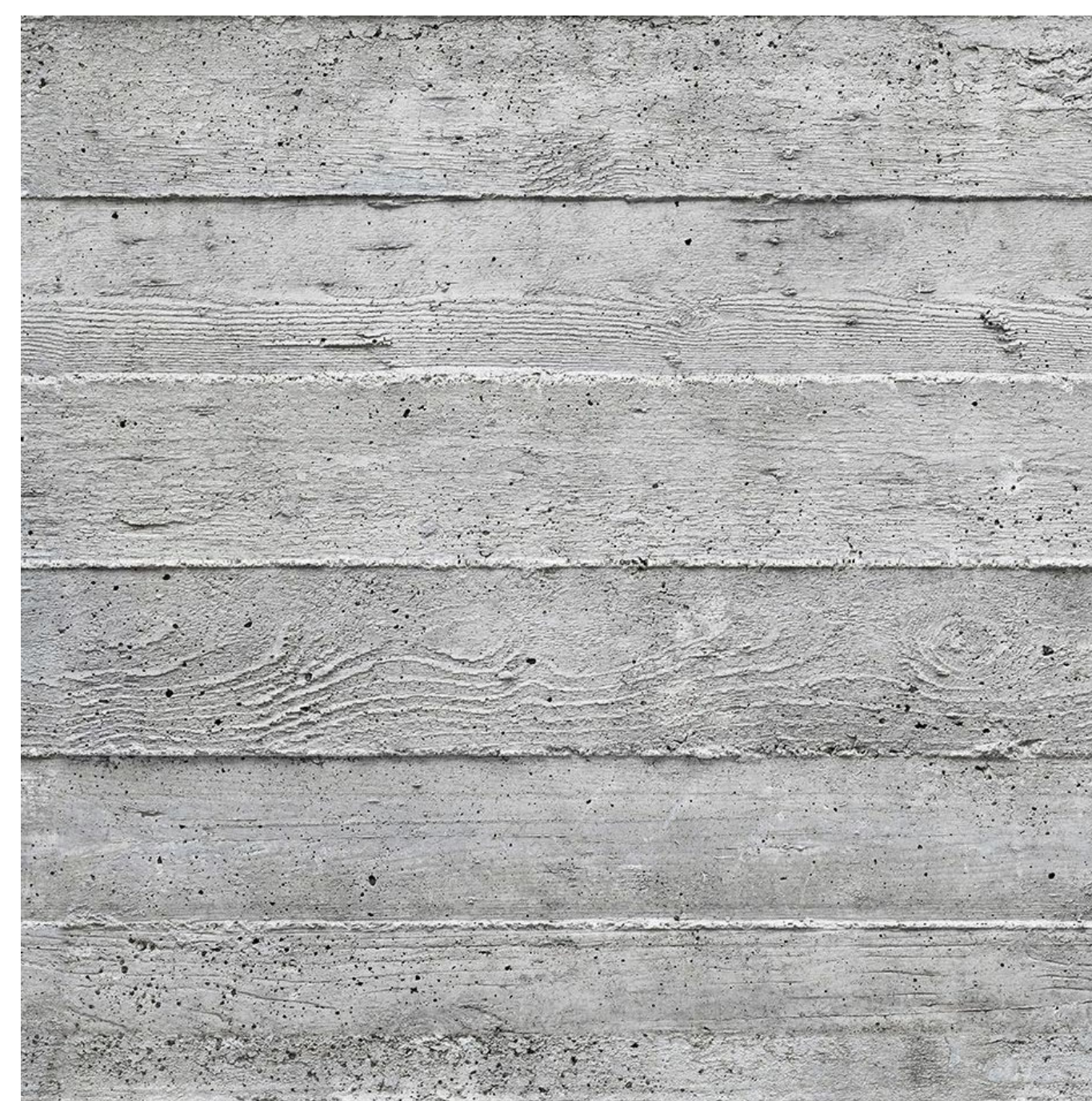
BOARD FORMED FINISH CONCRETE
