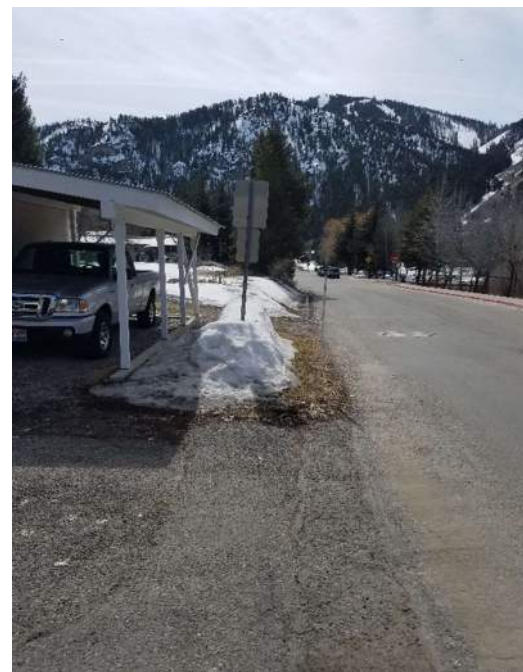
8th Street from Mid-Block Facing West- Carport Encroachment
