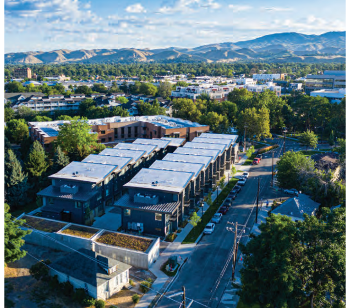
Ash + River Workforce Housing Boise, Idaho
