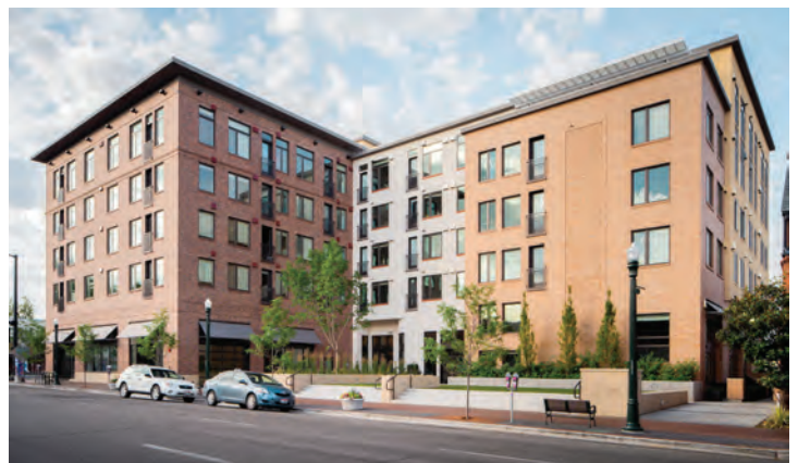
Ash + River Workforce Housing ( upper ) Boise, Idaho
