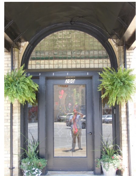
Door with fanlight. 200 N Main St
