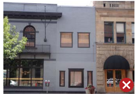
Inappropriate window proportion and detailing.
