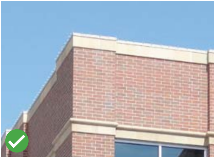
Acceptable parapet detail.
