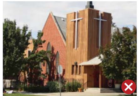
Inappropriate material selection.
