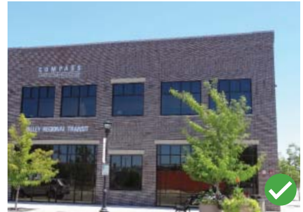
Appropriate use of brick.
