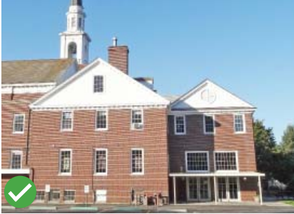
✓ Addition (at right) responds to existing form and materials.
