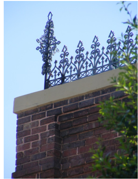
Architectural metal. 15 SE Court Sq
