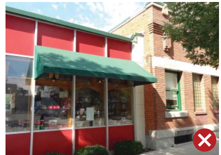
Inappropriate material selection.
