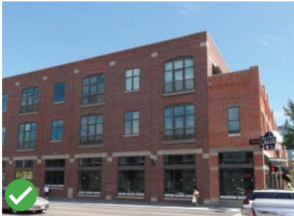
Appropriate alignment of original elements.
