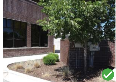
Acceptable screening of utility and garbage.
