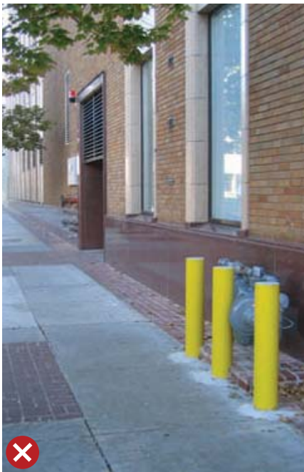
Utilities should not be located on sidewalk.
