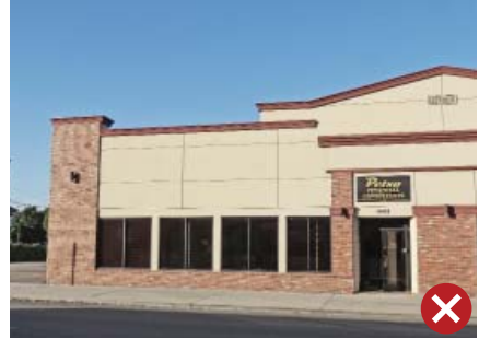
Inappropriate use of E.I.F.S.
