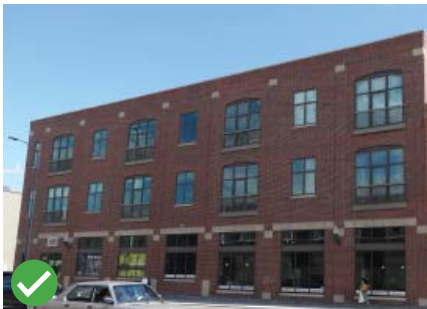
Appropriate segmenting of longer building facade.
