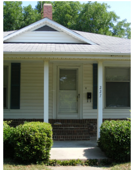
Gabled roof feature. 227 W Elm St
