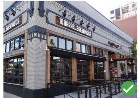
Appropriate bay in-fill. Appropriate materials.
