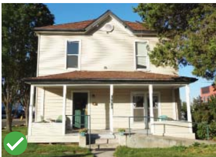
Acceptable ADA ramp addition.
