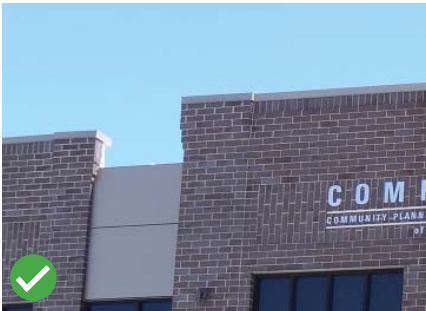
Acceptable parapet detail.
