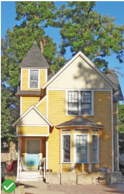
Addition preserves and relates to original house.
