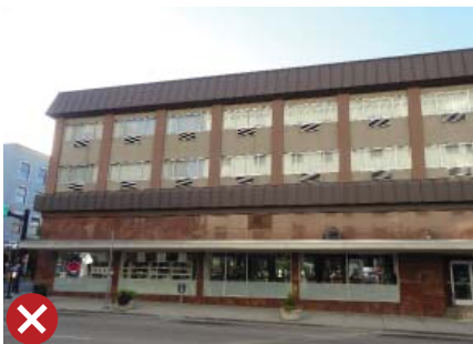
Inappropriately proportioned openings.
