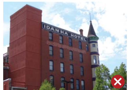
Exit stairway scale overwhelms historic facade.
