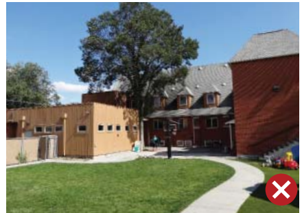
Inappropriate proportion, style, and material.
