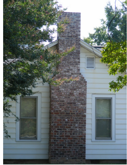
Chimney. 304 W Elm St
