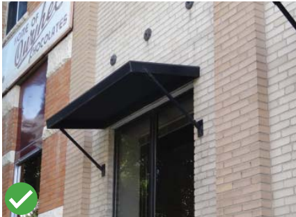
Compatible fixed shading device.
