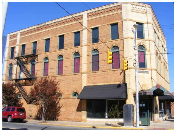
Exterior fire escapes. 200 N Main St
