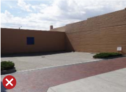
Inappropriate lack of screening.
