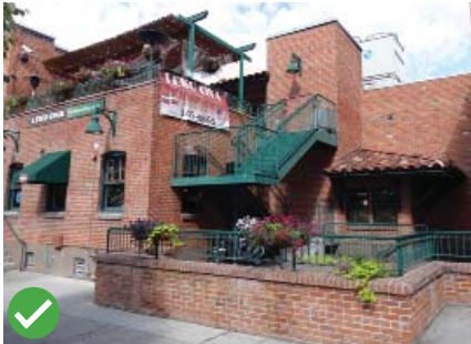
Compatible trellis, site walls, stairs, and awning.
