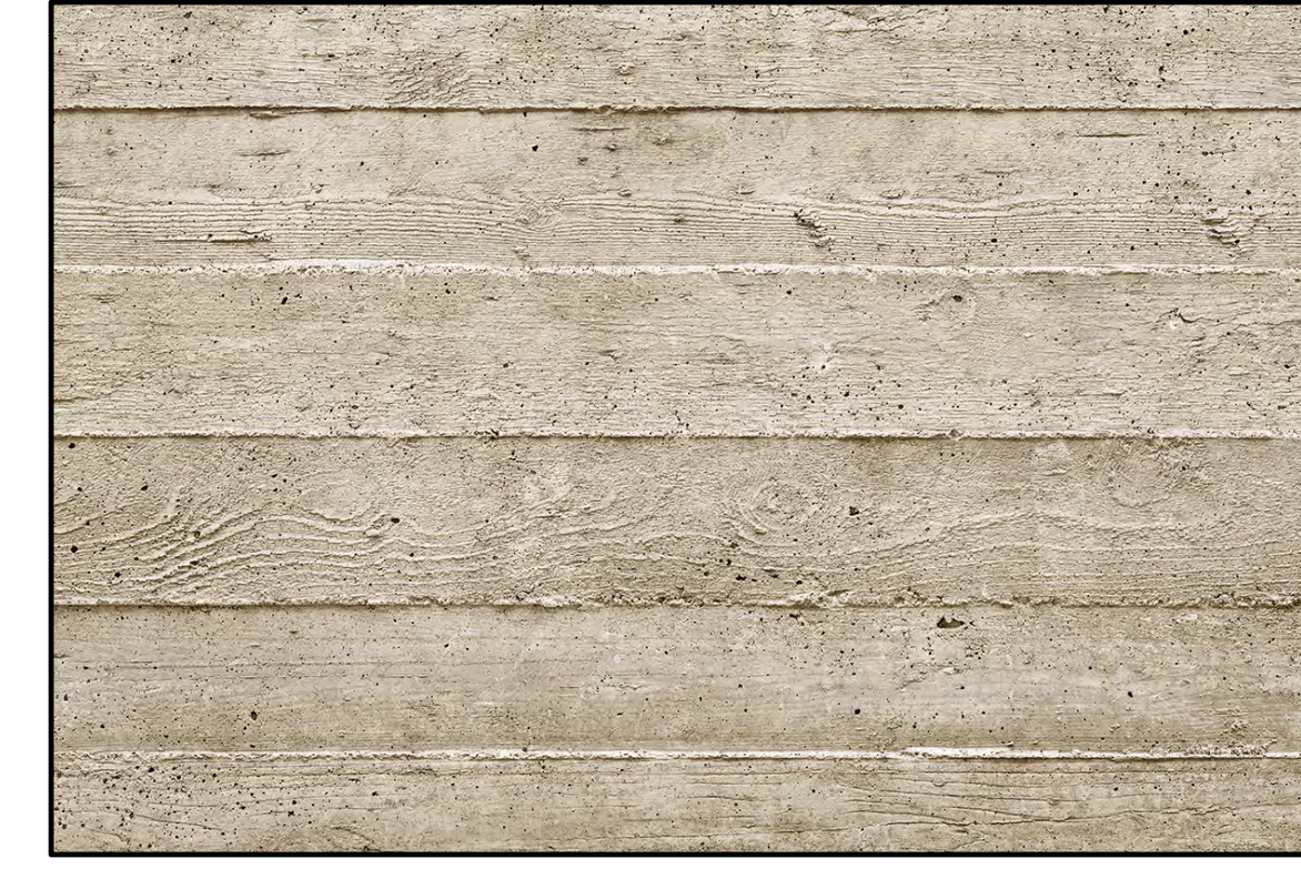
EXTERIOR FINISH 4 (EF-4): TINTED BOARD-FORMED CONCRETE
