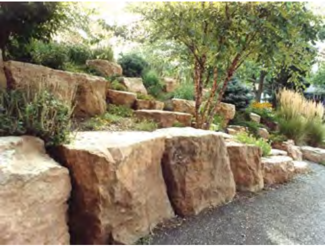
DRYSTACK BOULDER WALLS
