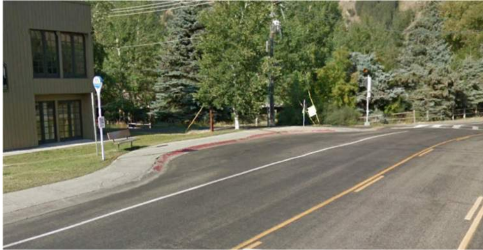
Figure 11: Existing Mountain Rides Bus Pullout. Source: Google Earth
