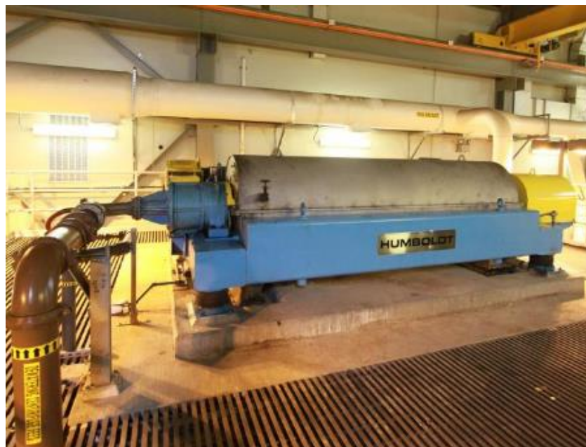
Figure 5-7. Centrifuge at Durham AWWTP in Portland, OR
