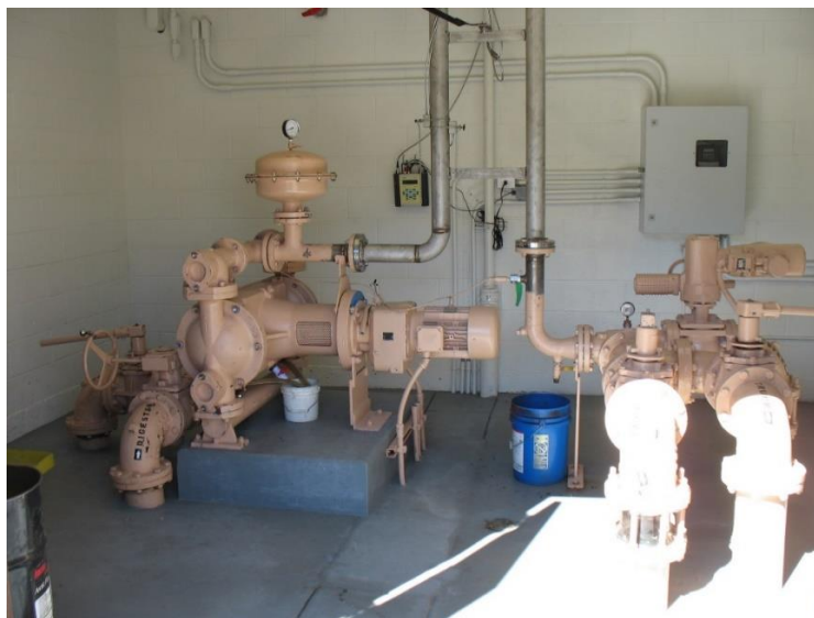
Figure 3-20. Biosolids transfer pump room
