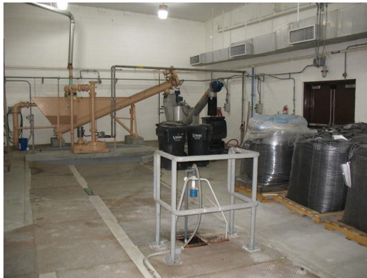
Figure 3-4. Grit chamber, conveyor, and washer room
