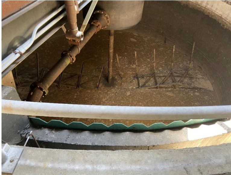
Figure 5-1. Existing gravity thickener
