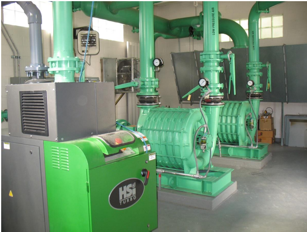
Figure 3-19. Digester blower room
