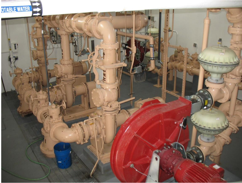
Figure 3-10. RAS and WAS pumping room
