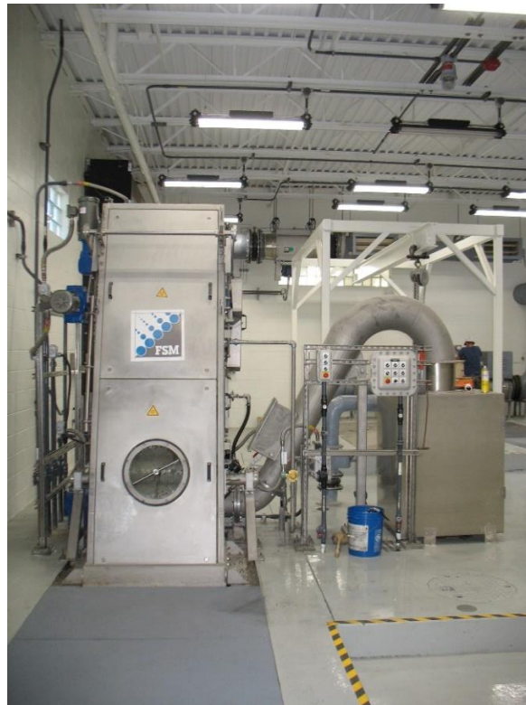
Figure 3-3. Perforated mechanical screen
