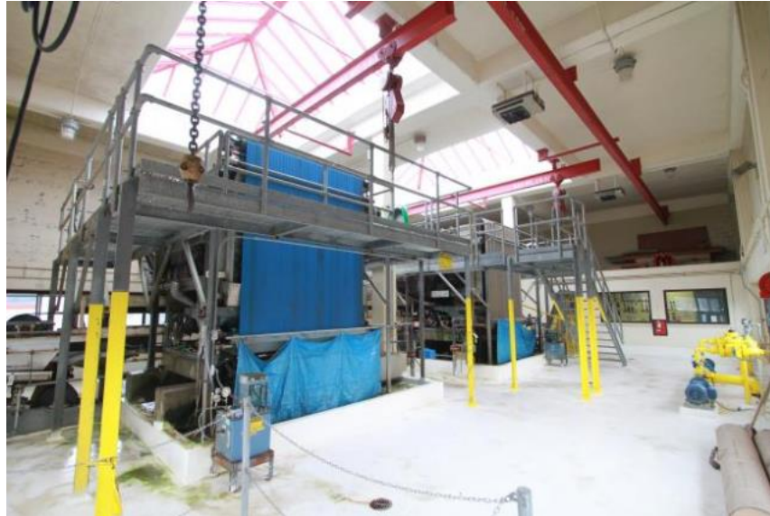
Figure 5-6. Belt filter press at the Newberg WWTP in Newberg, OR
