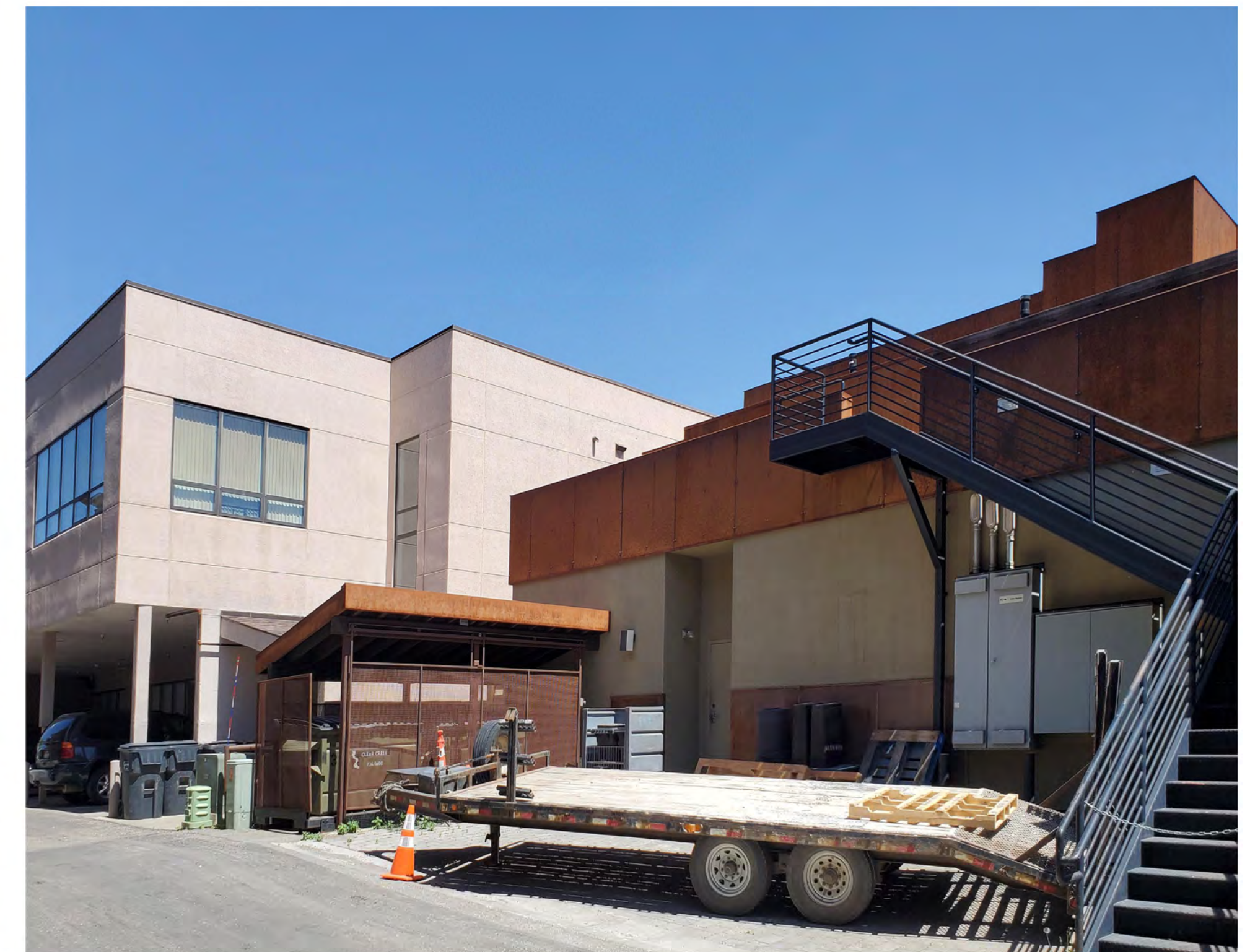
existing south west view
