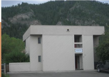
"Hyperborean Condo" Existing Structure on Site
