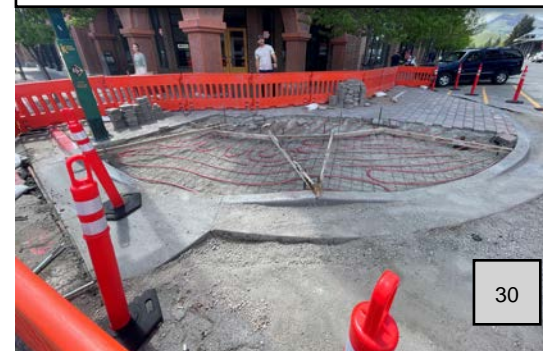
Example bulbout/ snowmelt construction
