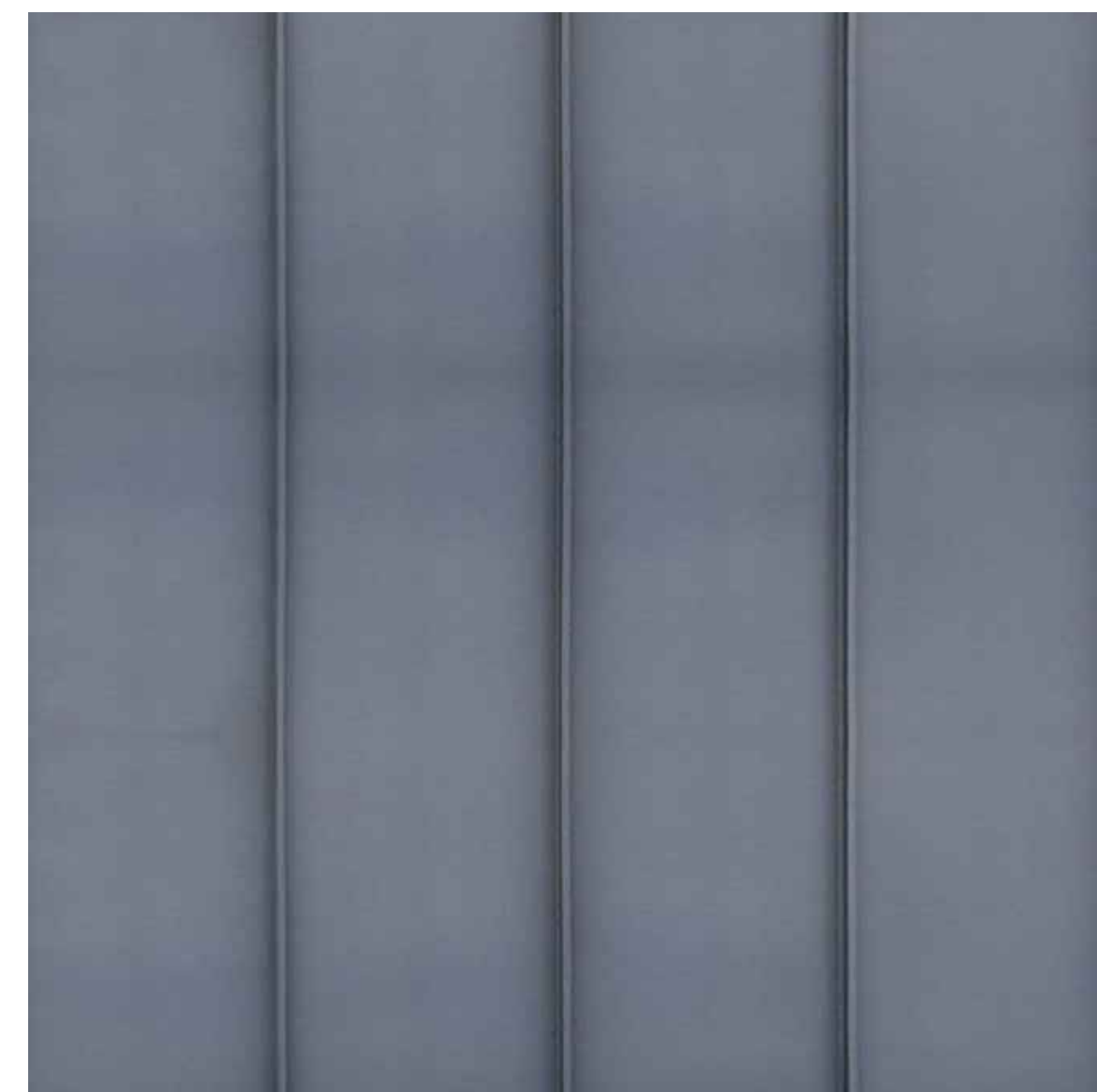
6) Zinc At chimneys & parapet caps
